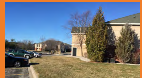
These apartments need sidewalks along the edge of the parking to eliminate pedestrian and vehicular conflicts in the parking lots
